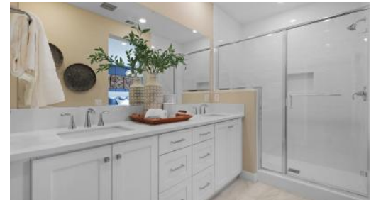
Framed shower enclosure with ceramic tile surround and tile floor
